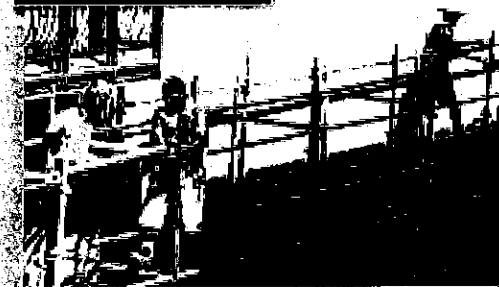
JJL Scaffolding - No fall prevention or dropped objects controls in place
